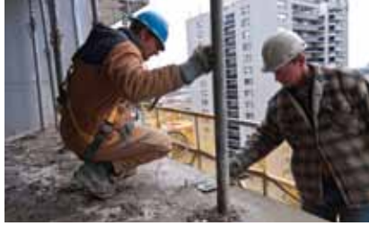
Refurbishing underway at Leslie York Mills
