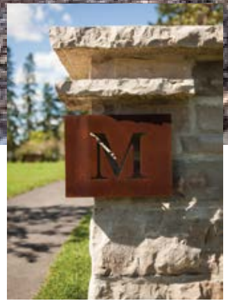
WELCOME SIGN This sign, made of Corten, a weathering steel that forms a stable rust-like appearance when exposed to the elements, welcomes homeowners and visitors. Its appearance is subtle and tasteful, in keeping with the community's village-like feel.
