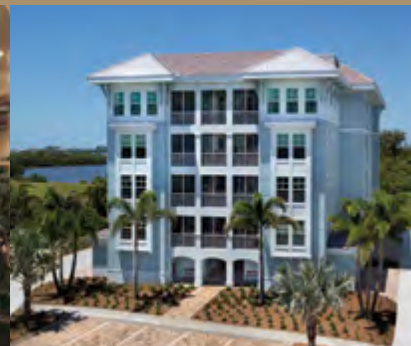
HARBOUR ISLE / Bradenton, FL
