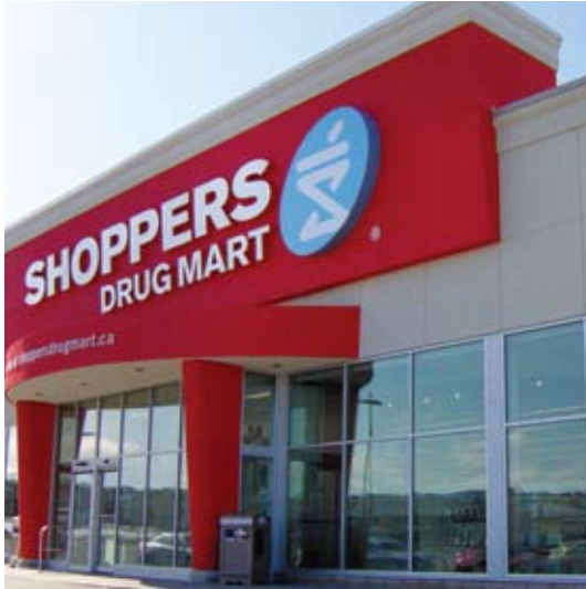
Clondike Crossing, Minto Commercial Properties Inc., Ottawa
