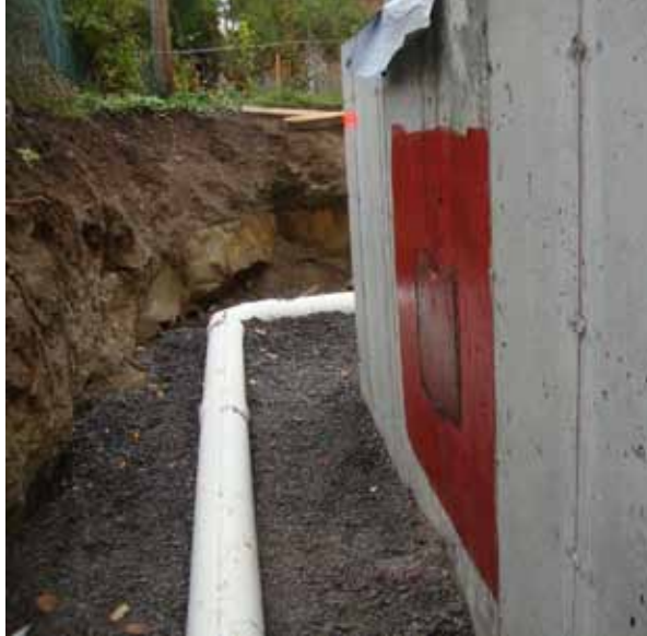
Photo: Earth Tube Pilot Installation
