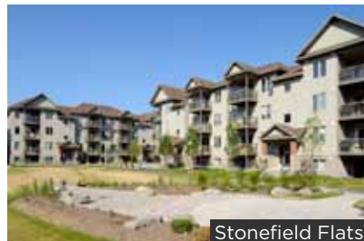
Stonefield Flats Drought tolerant plants Green plugs LEED® Canada for Homes community certification
