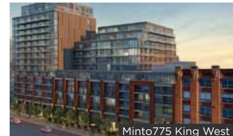
Minto775 King West 3L toilets Electric vehicle charging infrastructure
