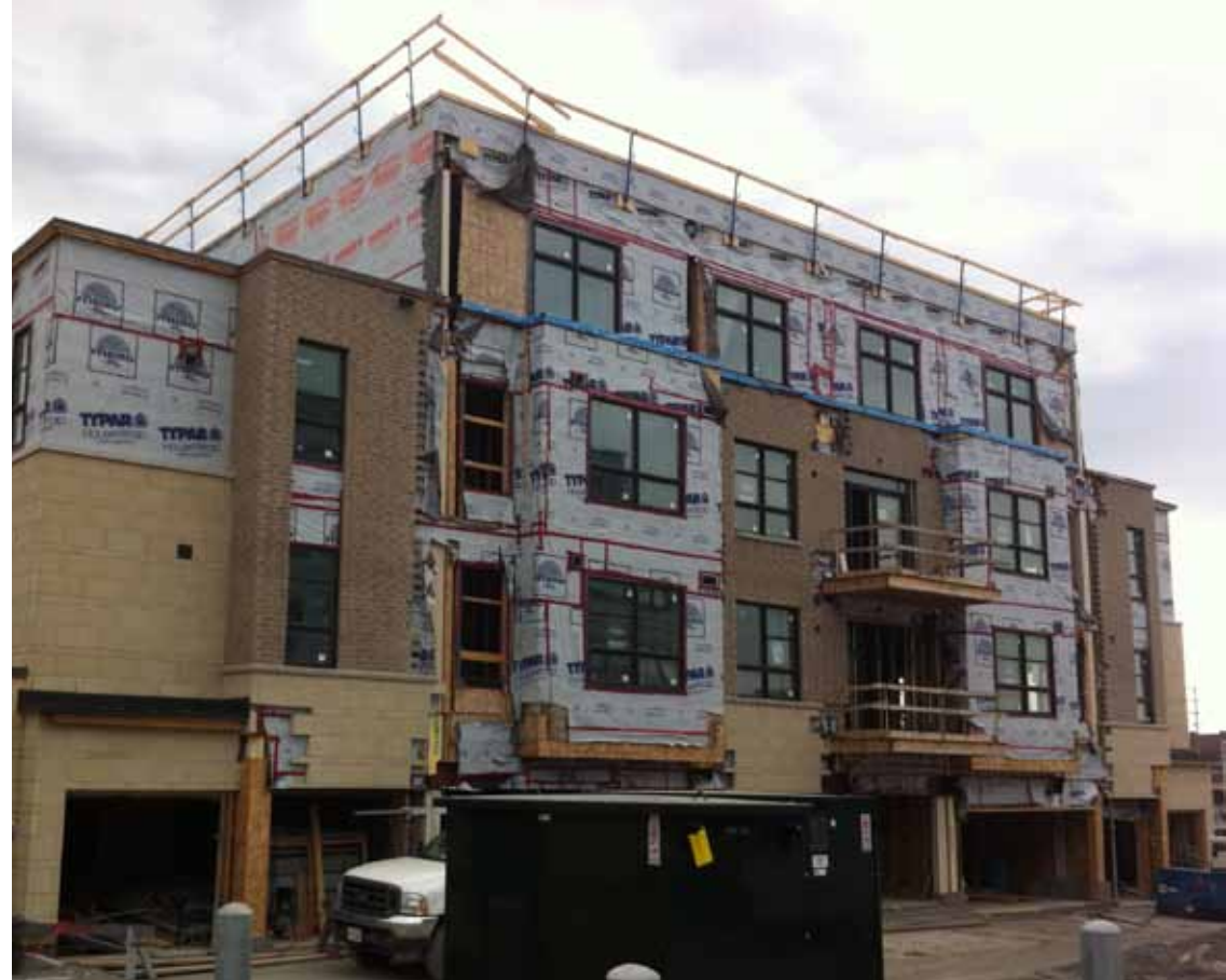
Photo: Construction of Minto Ampersand, Ottawa, ON
