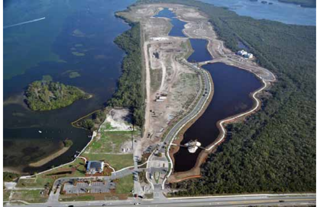
Photo: Harbour Isle, targeting LEED® certification, currently under construction, Anna Maria Sound, Florida
